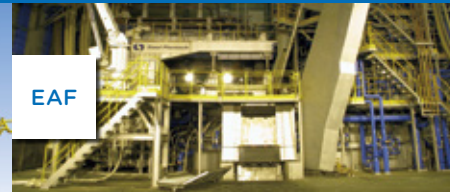
Ecological and Economical Arc Furnace (ECOARC™)
